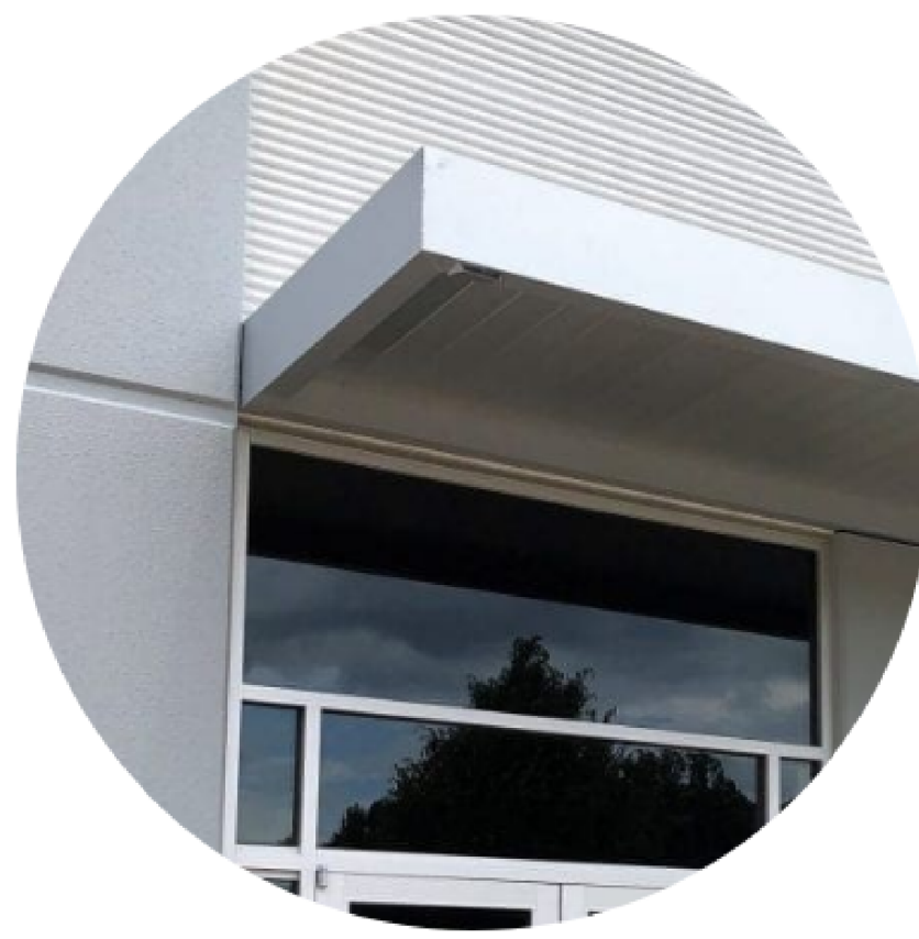
ALUCOBOND EYEBROW CANOPY PROJECTION
